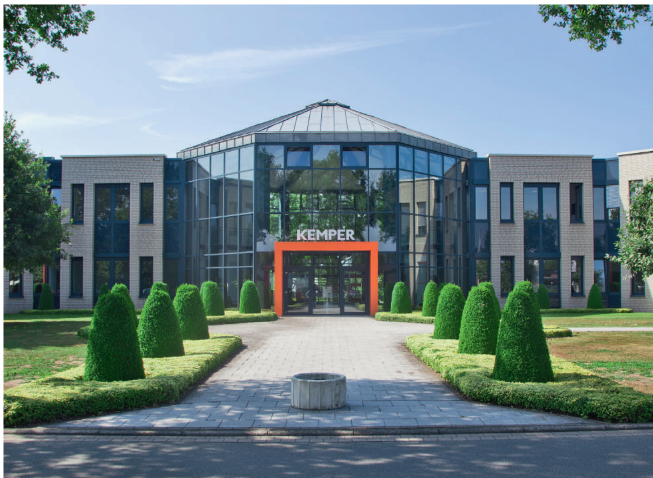
The KEMPER headquarters in Vreden, Germany.
